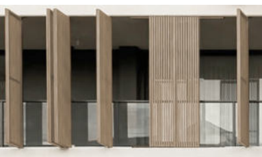
SCR7 | L02 BLDG D Bifold Screen Aluminium, Rectangular Sections Pale Timber-look Finish
